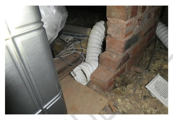
NON-FIRE RATED DOWNLIGHTERS ABOVE THE BATHROOM. THE ELECTRIC CABLES LOOK OLD.
