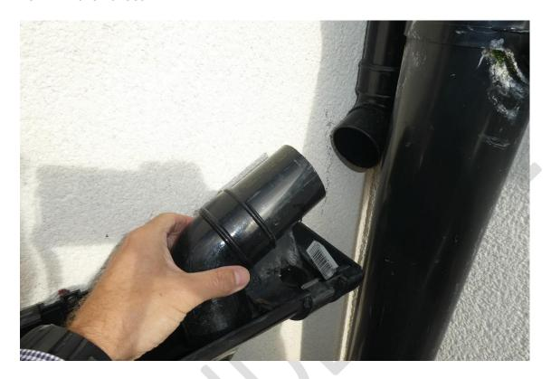
NEIGHBOUR'S OVERSAILING GUTTER AND OUTLET WITHOUT A DOWNPIPE.
